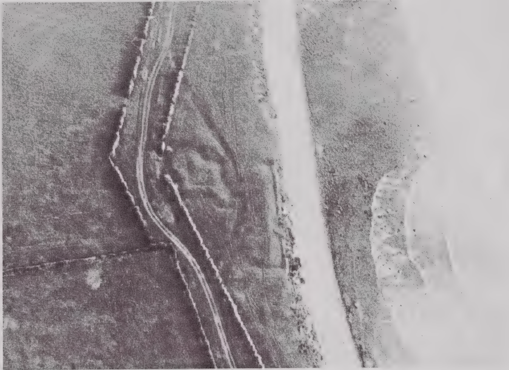
Fig. 16. Warea Redoubt. Aerial view to the south, 1975.
